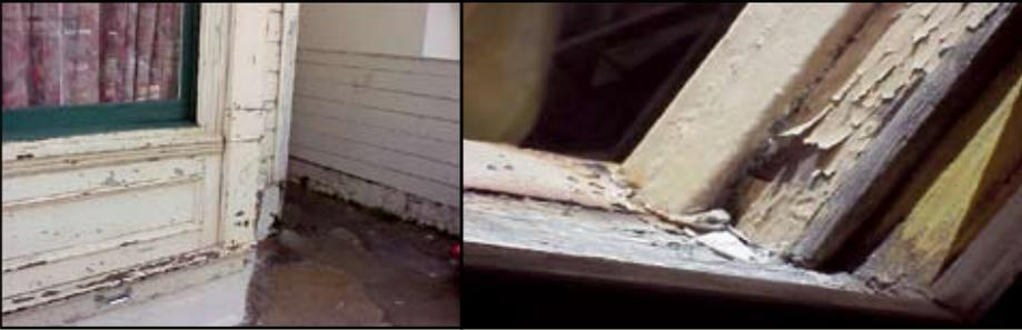
When property owners delay maintenance of their rental properties, older lead paint layers will degrade through peeling, chipping, chalking or cracking. Lead paint kept in poor condition releases lead dust particles.
